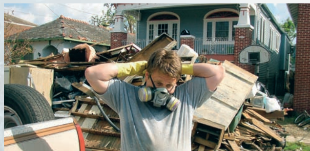
Pastor John Gerhardt, executive director of Urban Impact, prepares to enter his home to begin cleaning up. The pile of debris out front came from his first floor.
